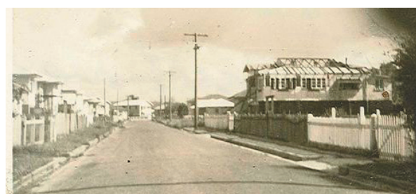
Figure 25: Roof Loss in Norman Street
