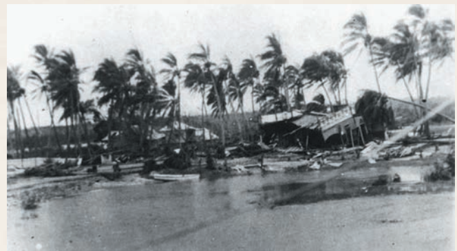
Cyclone damage along the Pioneer River, Mackay, 1918.
