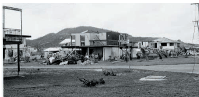
Figure 63: Damaged houses in Pallarenda, after Cyclone Althea. Source: CityLibraries Townsville Local History Collection
