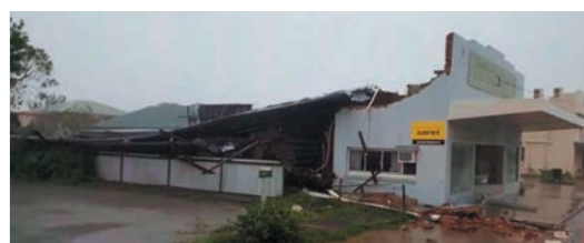
Figure 3: A badly-damaged plumbing business in Proserpine, 101km north west of Mackay. Source: ABC News
