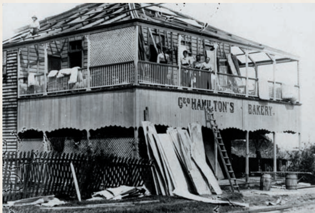
George Hamilton's Bakery damaged post impact.
