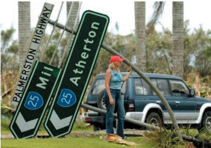
Figure 85: A road sign bent by the wind in Innisfail after Cyclone Larry in March 2006. Source: ABC
