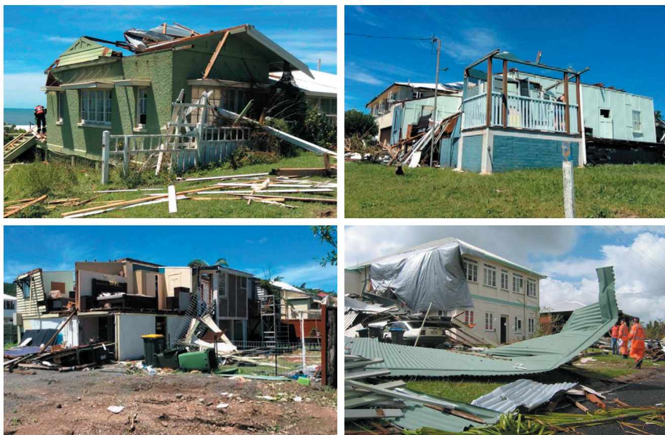
Figure 12: Damage to buildings in Yeppoon in the aftermath of Tropical Cyclone Marcia, 2015. Source: Queensland Fire and Emergency Services
