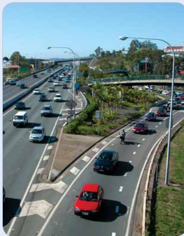
Motorway at Vulture Street, Brisbane Photo: Laurence Knight
